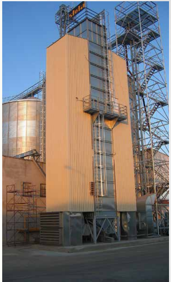
Project: Jevisovice Czech Republic Type: MDB-XN 1/13-SU Year: 2006 Product: maize Drying capacity: approx. 15,6 t/h from 35% to 15%
