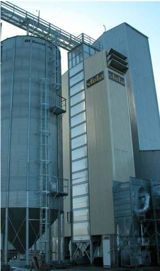
Project: WMW Serbia and Montenegro, Melenci Type: MDB-XN 1/15-SU Year: 2006 Product: maize Drying capacity: approx. 20,0 t/h from 32% to 14%
